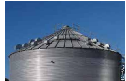
Silos with ventilation units
